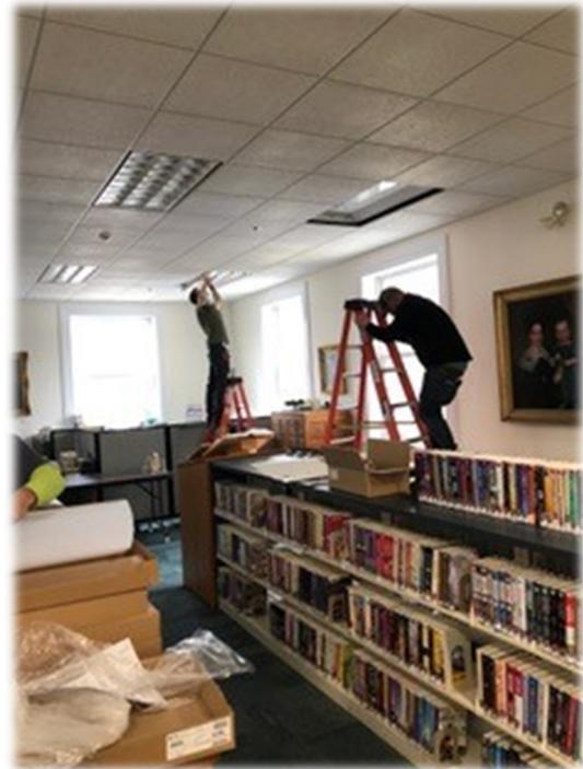
*New energy efficient ceiling lights being installed*
