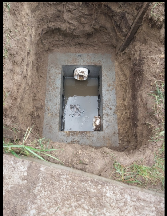
DISTRIBUTION BOX IN SEPTIC SYSTEM
