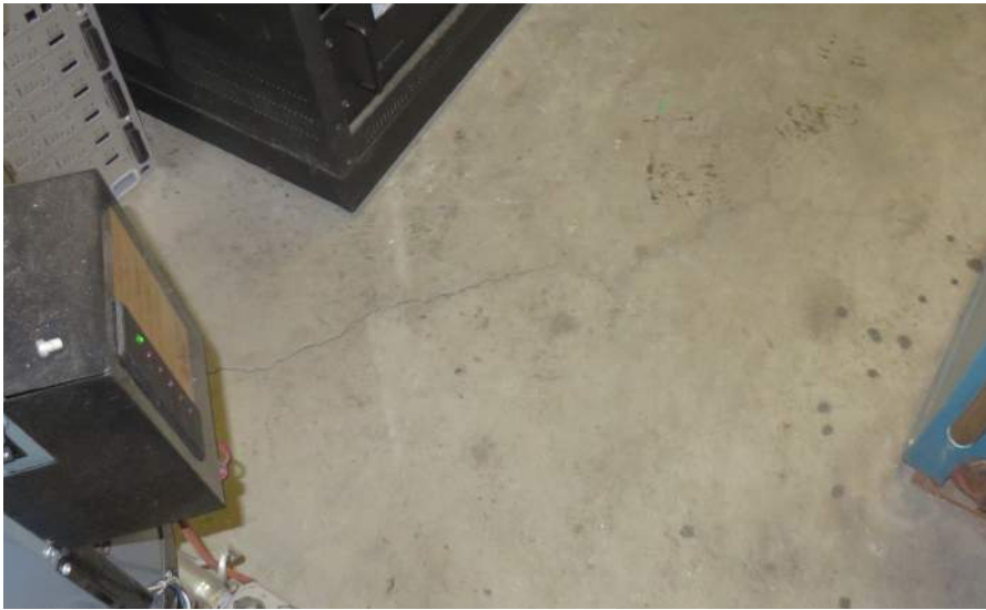
4 - Concrete slab-on-grade hairline cracks - Police Department
