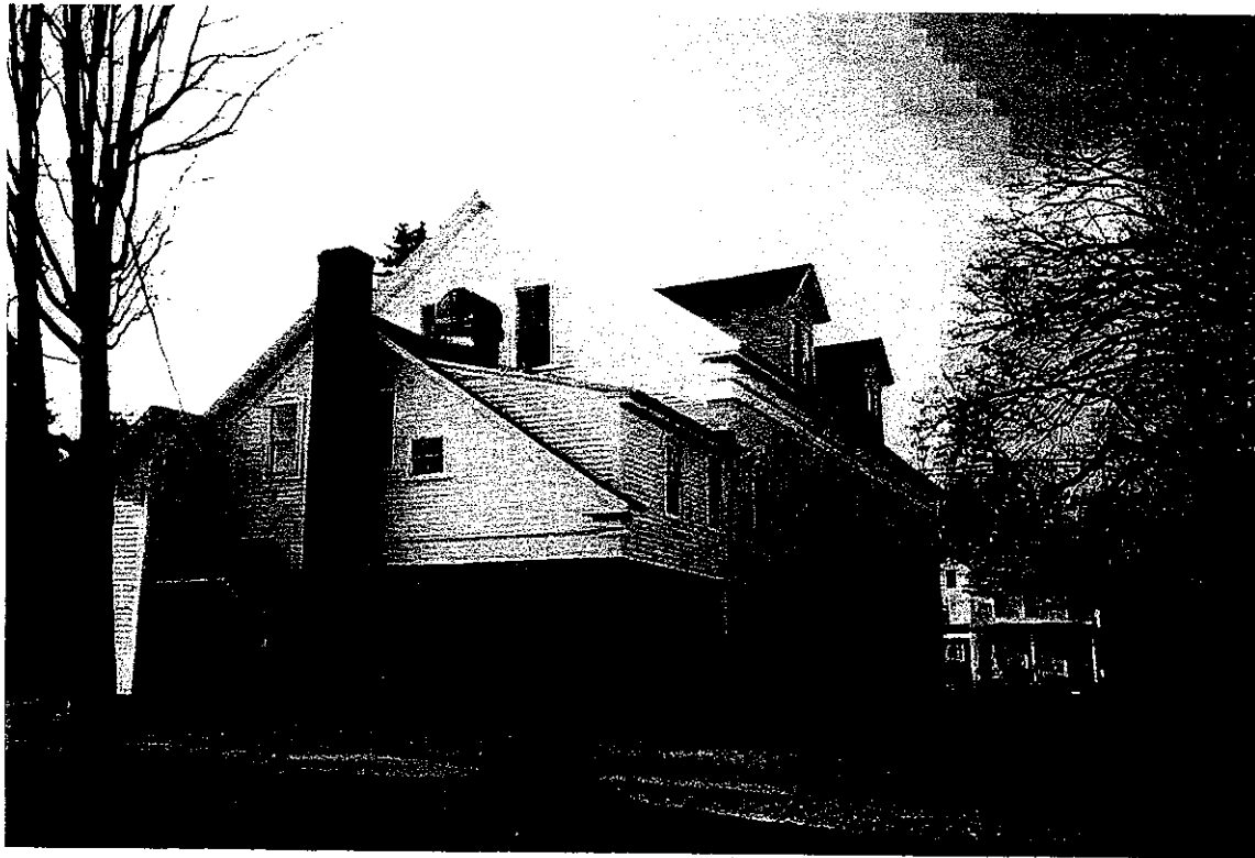
Town Hall – Rear View North. New Addition in place of 1 1/2 Story Element could include New Accessible Entrance and Elevator.
