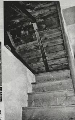
The steep steps that lead up to the attic.
