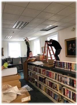
New energy efficient ceiling lights being installed
