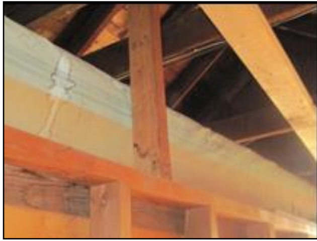
Ceiling beam – second floor
